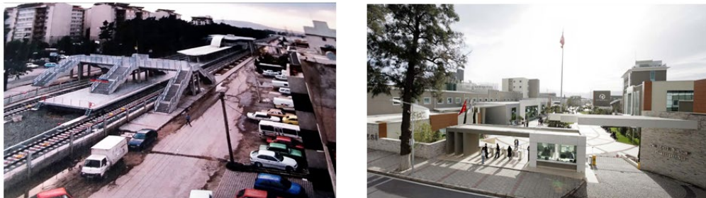
Figure 4.13: Bornova Metro Station in 2000 (on the left) -Yaşar University Campus, 2007 (on the right)
